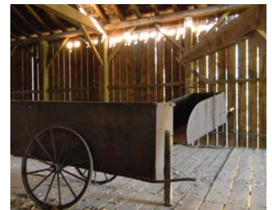
The Buckeye Furnace charging shed, with its giant scoop, was used to feed the smelting fires from above.
